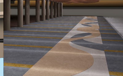
Colored concrete shared use path sidewalk
